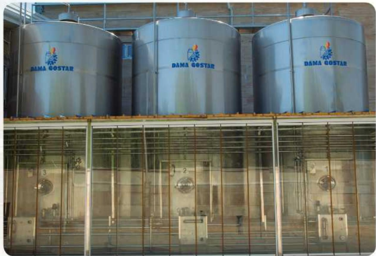
Tanks to the high efficient heat exchanging parameter the reservoir tanks with different capacity from 10.000 lit to 70.000 lit are well designed for milk , juice and food grade oils storage which in turn may be set up either vertically or horizontally based on the other lined-in machines.
